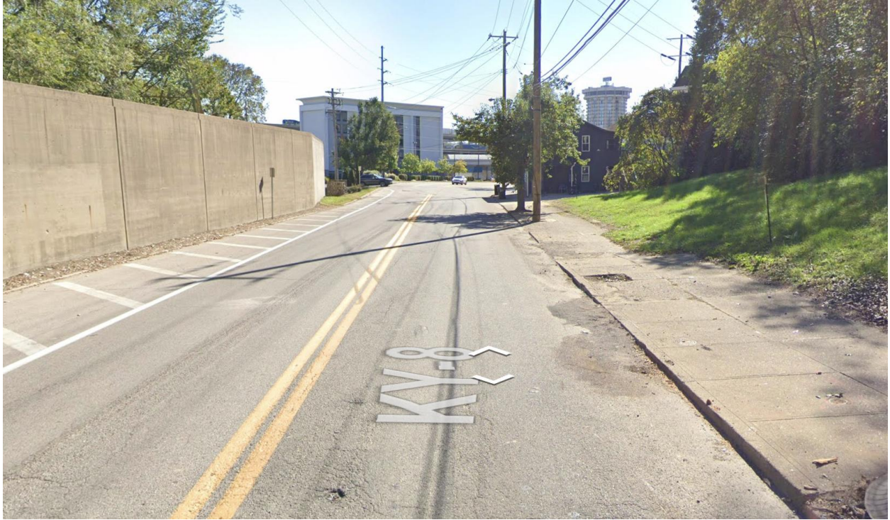
View of Crescent Ave. from the north end looking east. Note the floodwall on the left.
