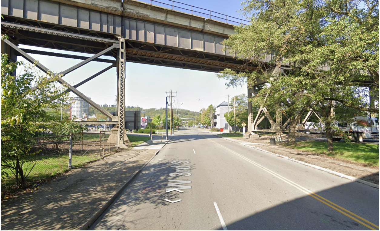
View of the railroad bridge area over West 3 rd Street, looking west.
