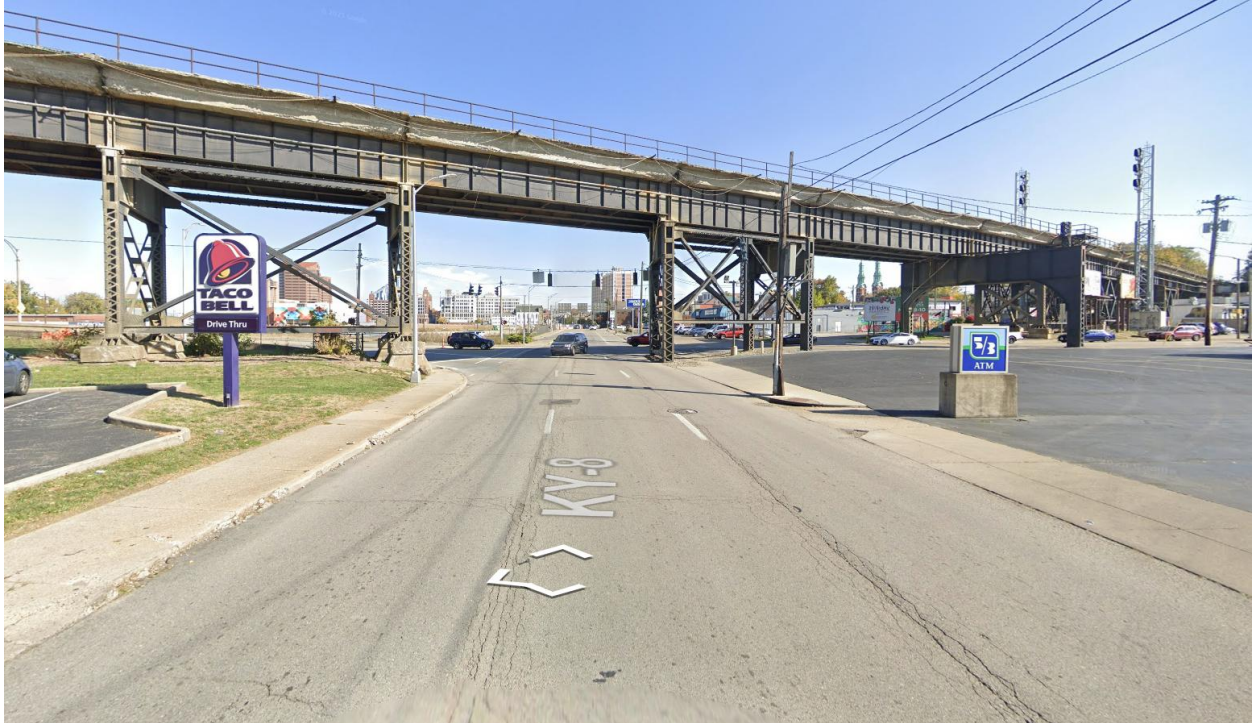
Middle of Area 3 looking east at the Rail overpass and intersection with Main Street.
