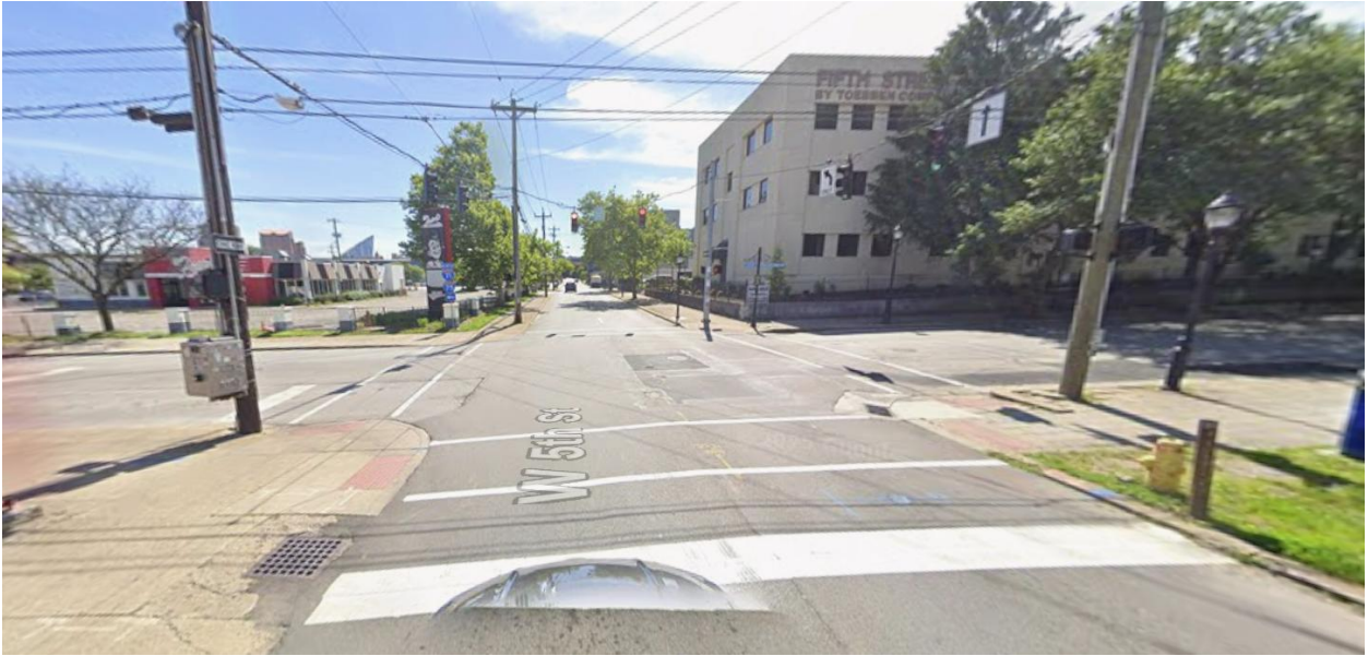
Area 4 looking east at the West 5 th Street/Philadelphia Street intersection.
