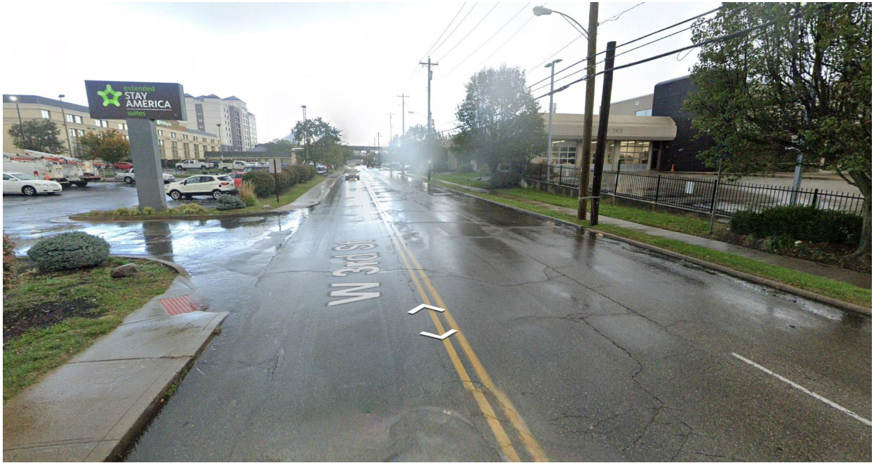
West end of Area 2 looking east on West 3 rd Street.
